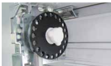
Fix the drive plate on the gear and secure.
