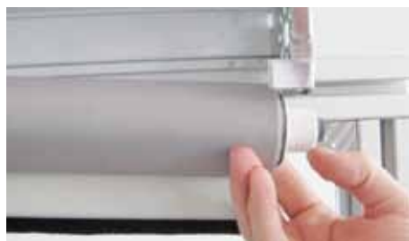
Clip the spring shaft bearing in the box
