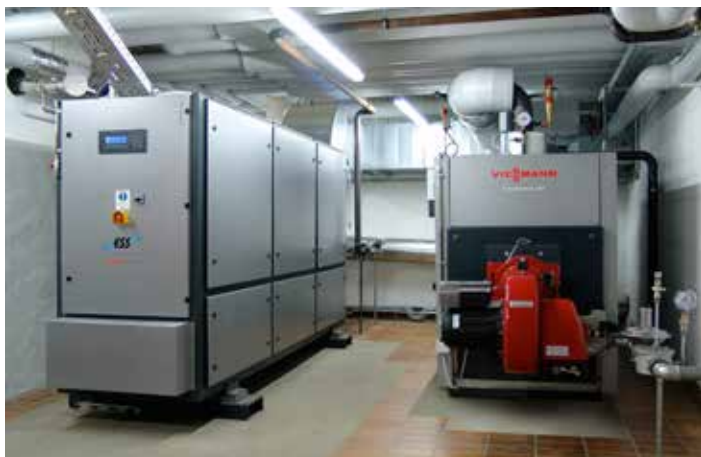
GEIGER cogeneration unit and peak load boiler
